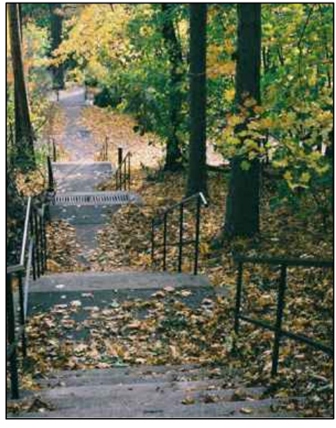
Direct route – stepped path with handrails
